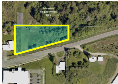
North Fork of Baker Creek earthen dam on city property
